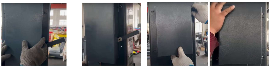
Feed the long end of the cable through the cable tensioner
